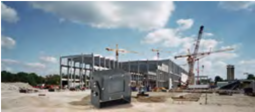
Construction machinery and cranes
